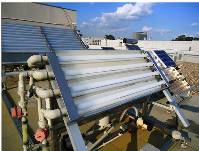
**Fig. 1.** Solar Pilot Plant with CPCs where the  $\text{TiO}_2$ -photocatalytic treatment of the WWTP effluent was performed.
